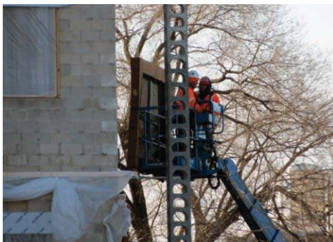
Windows being delivered to second floor.
